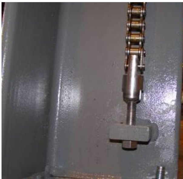
Figure 22 Connection to Lower Lug – Inner Chain
